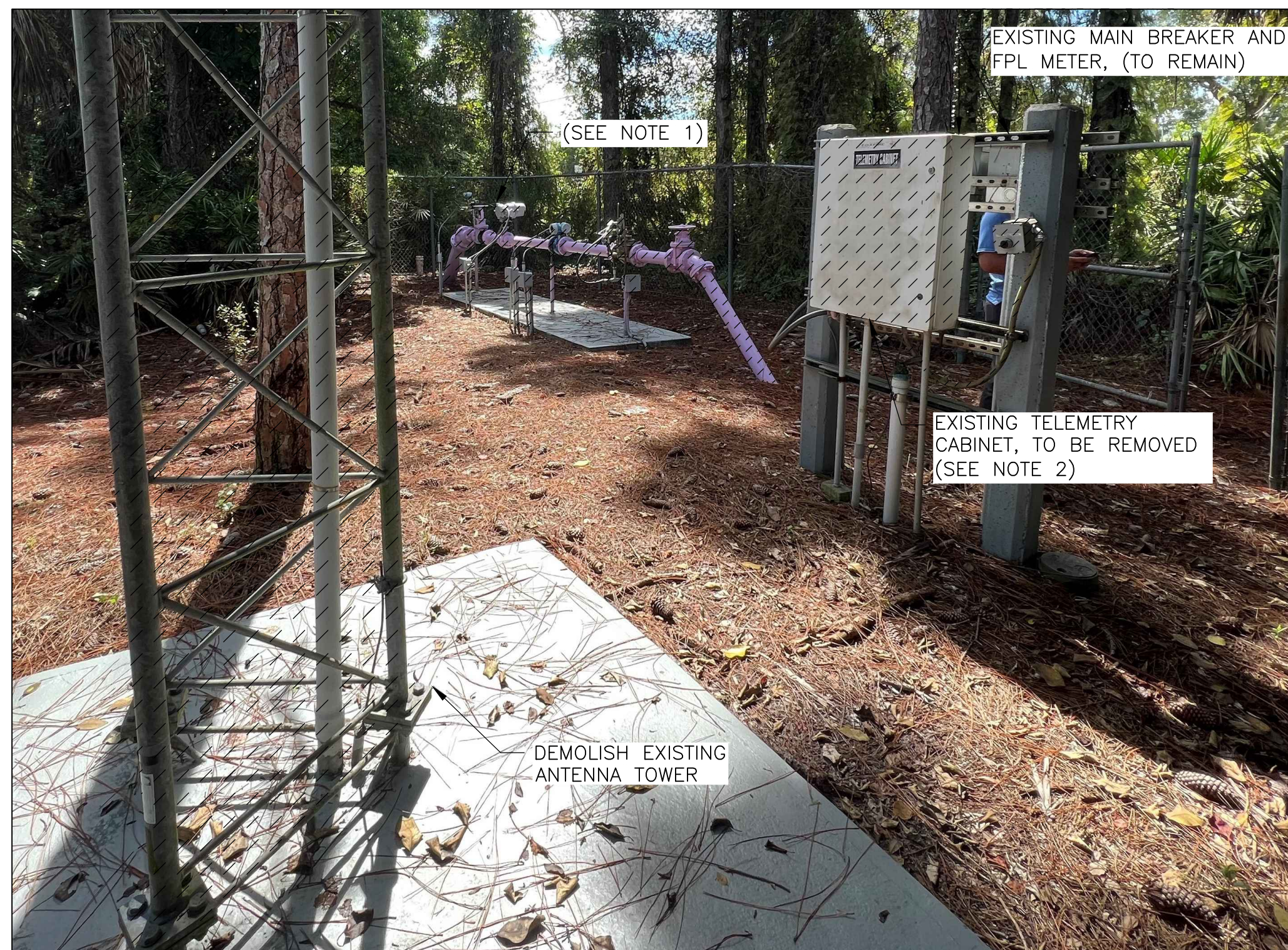
FOXFIRE 9 OUTFALL PHOTO NTS
