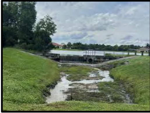
PHOTOGRAPH #01: A-17 WATER CONTROL STRUCTURE, FACING WEST
