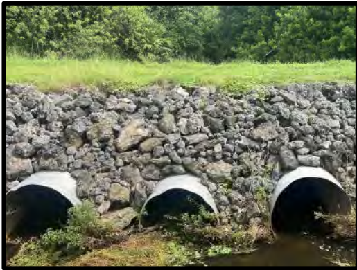
PHOTOGRAPH #03: A-18 CULVERTS, FACING EAST
